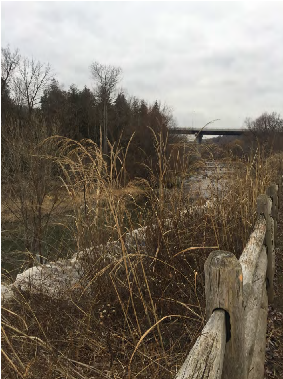
Highland Creek looking upstream to the Morningside Avenue bridge.
